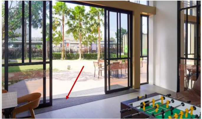
Figure 5.35: Accessible Entrance Threshold with Recessed Entrance Mat
