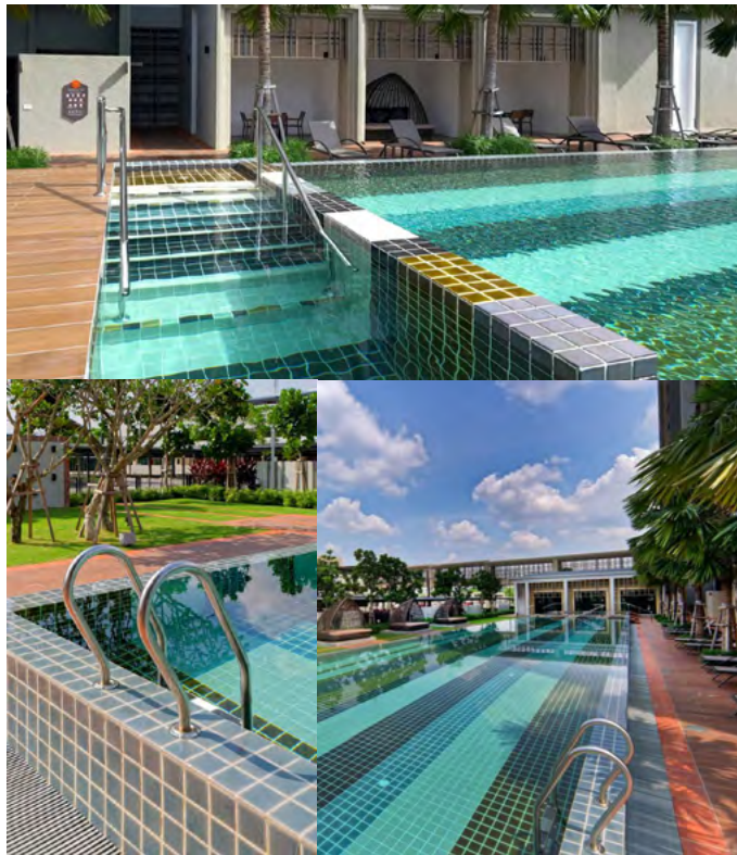
Figure 5.33: Accessible Water Entry with Safety Elements
