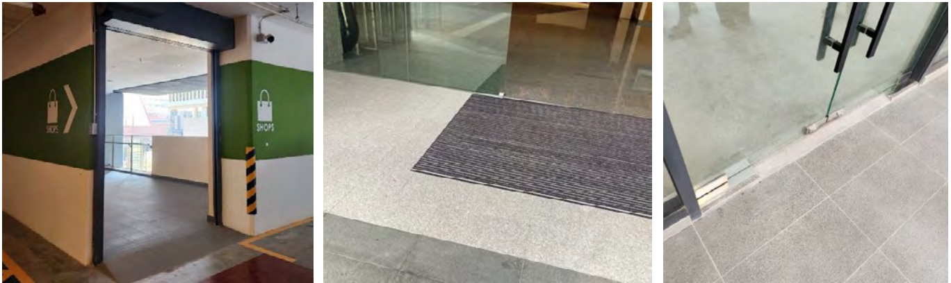
Figure 5.44: Seamless and Step-Free Access from the Car Park to Retail Areas and Outlets
