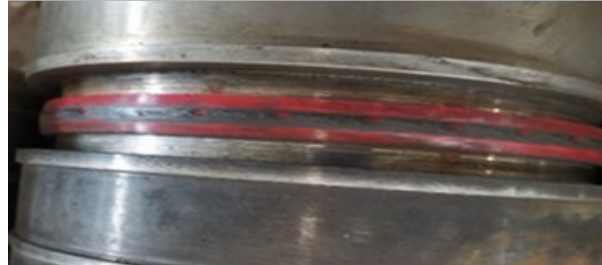
Figure 19.2: Example of seal failure
